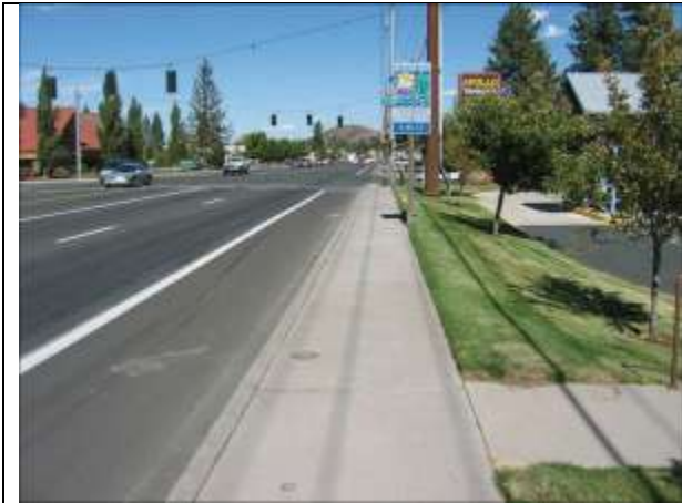
Figure 36. An example of a multilane arterial with a typical six-foot sidewalk and no buffering other than the bicycle lane. Pedestrians in such instances feel exposed to traffic, unsafe, and uncomfortable. Image: Freedman Tung & Sasaki
