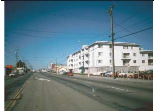
Figure 31. An apartment building inserted onto a corridor without compatibility with adjacent commercial uses, lacking buffering to arterial traffic, and displaying an unappealing ground-floor façade of parking garage grillwork. Image: Freedman Tung & Sasaki
