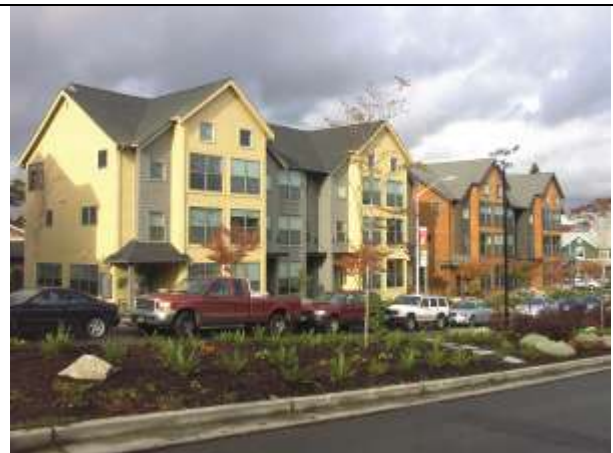
Figure 35. Rainier Vista, a new corridor housing development along a light-rail line in Seattle, Washington, uses a consistent set of features with variations—gable and sloping roofs with common slope and orientation, window types and sizes, and different cladding and color palettes.
