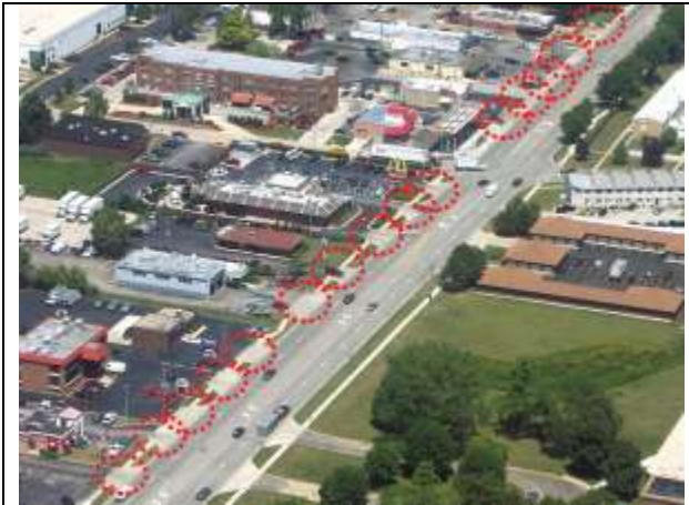
Figure 45. A five-lane strip corridor in northern New Jersey with small commercial uses and frequent driveway curb cuts, each circled in red, accessed by a two-way center left-turn lane. Image: Microsoft Virtual Earth
