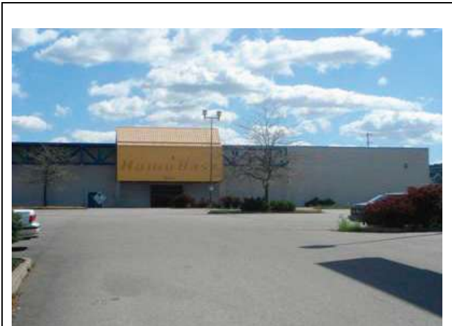
Figure 13. Disinvestment along the strip affects properties at all scales of development. Image: Freedman Tung & Sasaki
