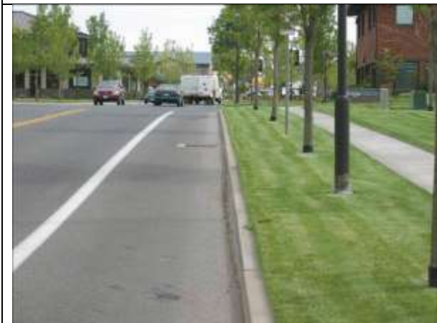
Figure 37. The addition of a planting strip with trees in between a similar sidewalk and bicycle lane substantially improves the comfort of the walking environment and the character of the street. Image: Freedman Tung & Sasaki
