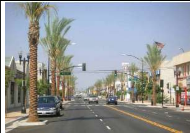
Figure 38. This right-of-way that was restructured to better support the downtown and introduces trees into the parking lane along the downtown segment (Whittier Boulevard Improvements, City of Montebello, California). Image: Freedman Tung & Sasaki
