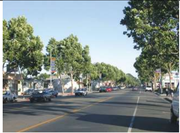
Figure 30. Today, this segment of East 14th Street has been restriped for three vehicle lanes and bicycle lanes in each direction. A continuous tree planting between the sidewalk and curb makes walking more comfortable and dramatically increases the corridor's appeal for mixed-use development. This was a capital improvement recommended in the North Area Specific Plan and Revitalization Manual, City of San Leandro, California. Image: Freedman Tung & Sasaki
