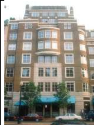
Figure 51. An urban apartment building with no setback and a shared lobby entrance built along the edge of the sidewalk. Image: Freedman Tung & Sasaki
