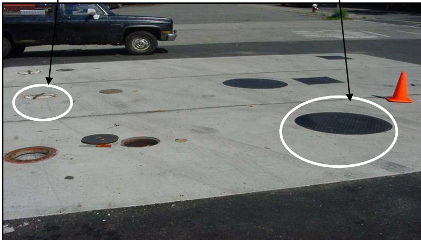
View of sump lids
