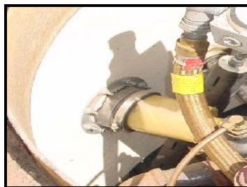
Sump penetration seals in good condition
