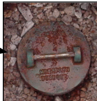
Closeup Of Extractor Port
