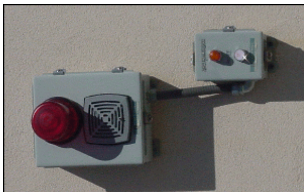
Sample Overfill Alarm
