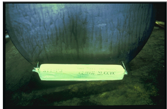
Sample Galvanic (Sacrificial) Anode
