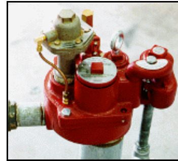
Sample STP Head With LLD
