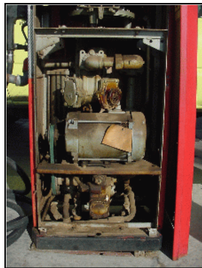
Example Of A Suction Pump Inside A Dispenser
