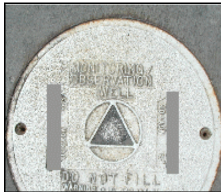
Sample Monitoring Well Cover
