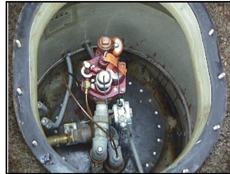
Sample STP Head In A Sump On Top Of A Tank
