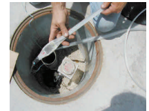
Interstitial monitoring sensor
