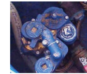
Submersible turbine pump without a LLD installed
