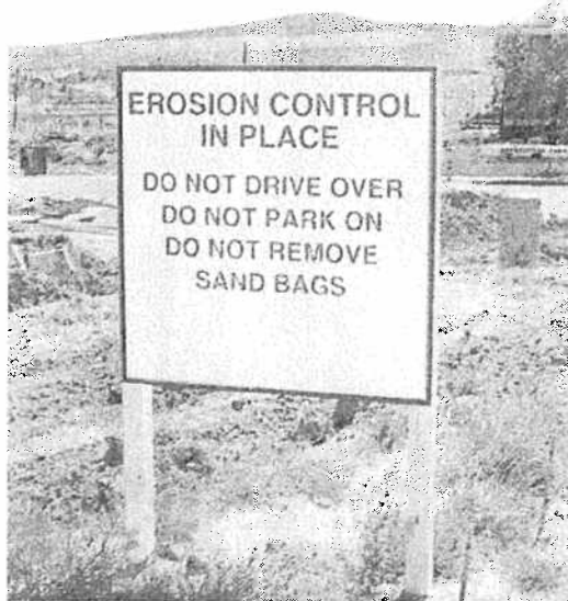
Figure 4. Use signage to help educate construction staff.
