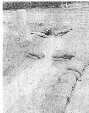
Figure 5. Make sure storm drain inlets are protected.
