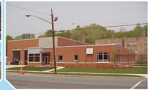
Site reused as a firehouse
