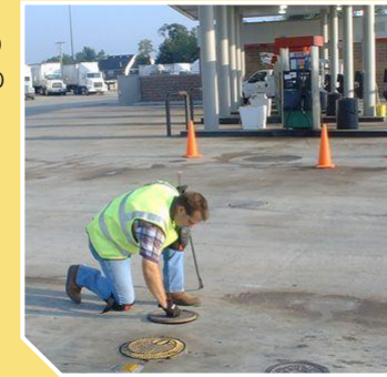
Inspecting a spill bucket
