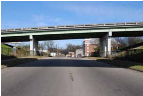
Figure 39: Existing view looking north along Holt Street.
