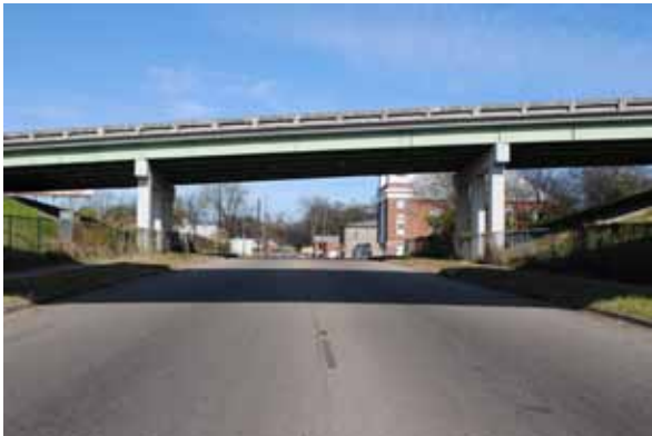
Figure 37: Existing view looking north along Holt Street.
