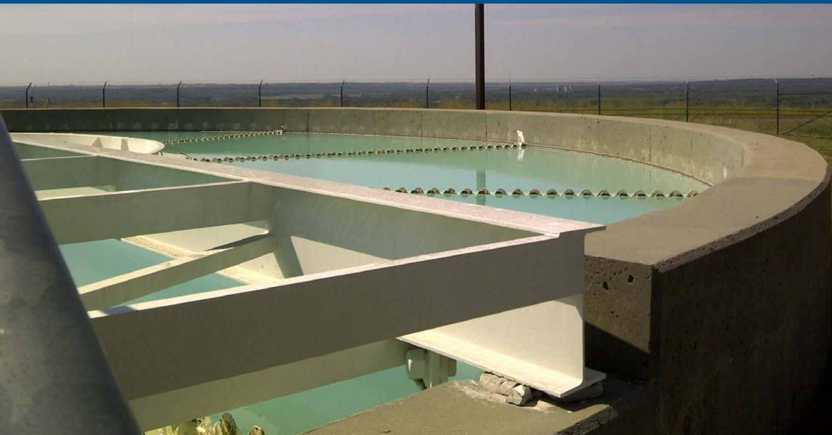
One of two waste water treatment facilities at Ft. Riley, KS.
