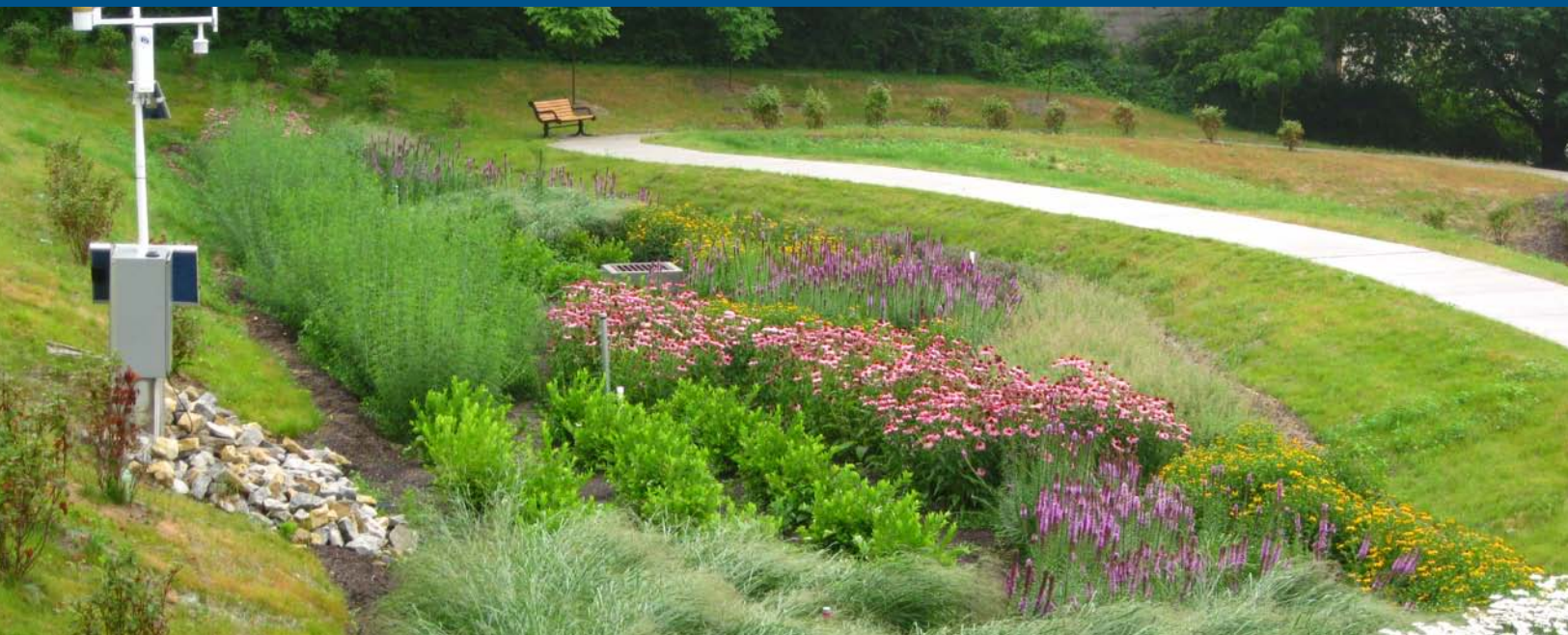
Rain garden pilot project with monitoring equipment at the St. Francis Court Apartments in Cincinnati.
