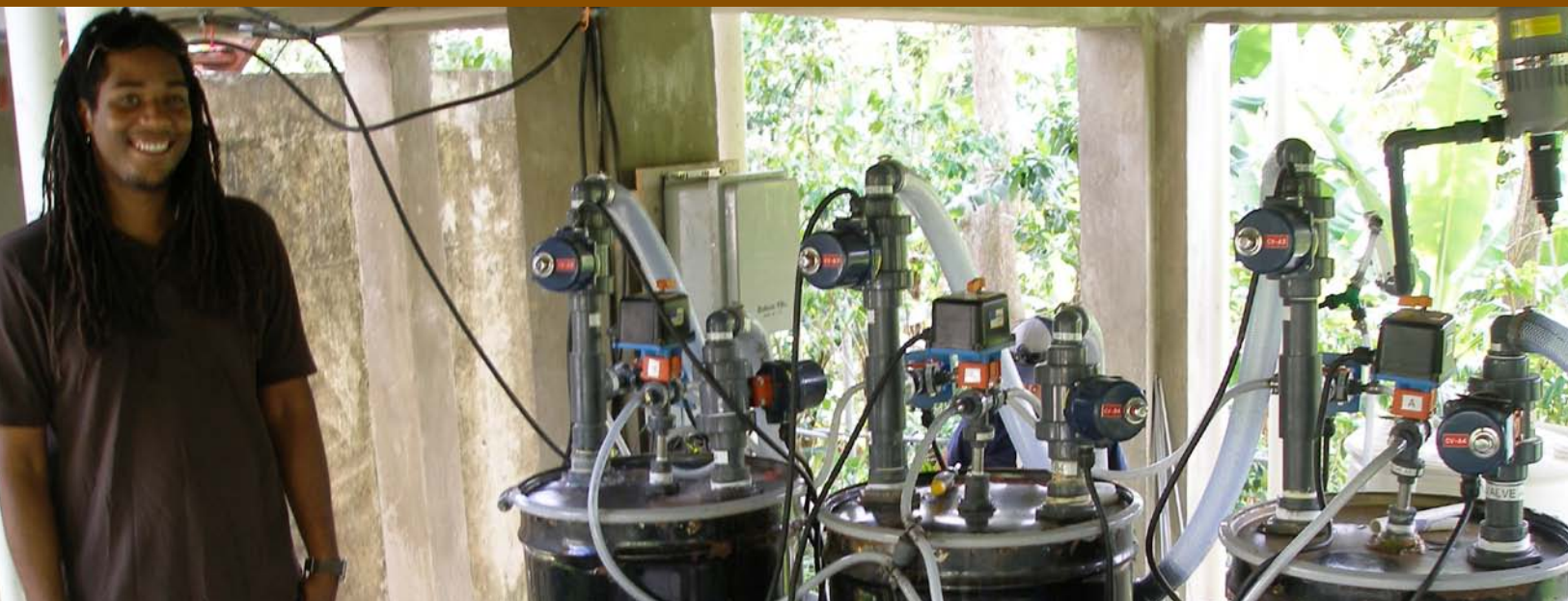
Two 55 gallon drums (in series) for sand filtration are always in service while the third is undergoing backwash. Daniel Concepcion, a University of Puerto Rico student, completed his Masters Degree based on these drum sand filter studies.
