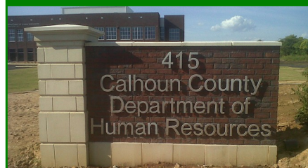
AFTER: The new DHR building completed in Oct 2012
