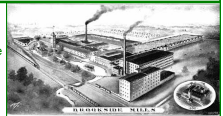
BEFORE: Brookside Mill, cir 1880s
