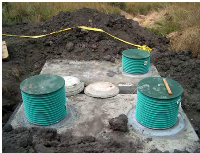
Installation of an advanced treatment system.
