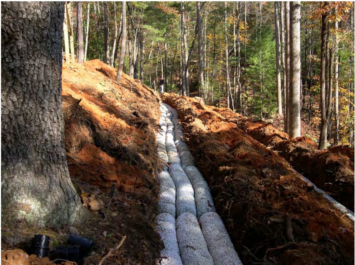
Non-gravel systems, like this one on a slope, account for half of the onsite systems installed in North Carolina. Photo: Department of Natural Resources, North Carolina.
