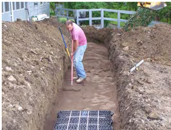
Installing a treatment system. Photo: Florida Department of Health.
