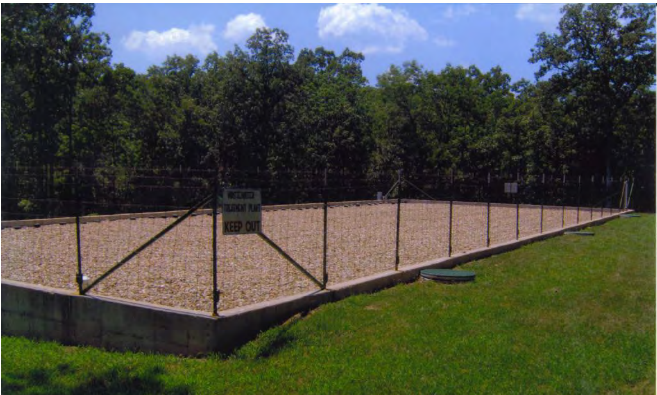
The Water Supply District serves as the RME in Phelps County, Missouri. The district owns and operates eight recirculating sand filters.
