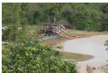
Figure 7. Fresh Water Hydraulic fracturing Pond
