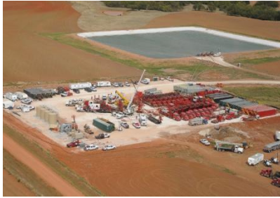
Figure 8. Fresh Water Hydraulic fracturing Pit
