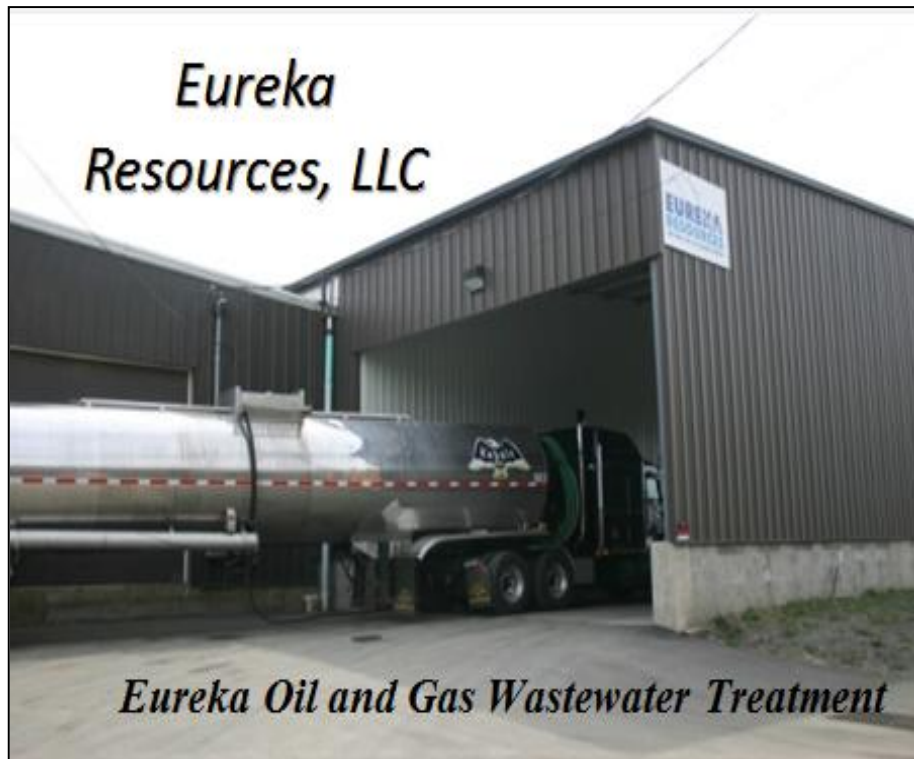
Figure 1. Eureka Oil and Gas Wastewater Facility
