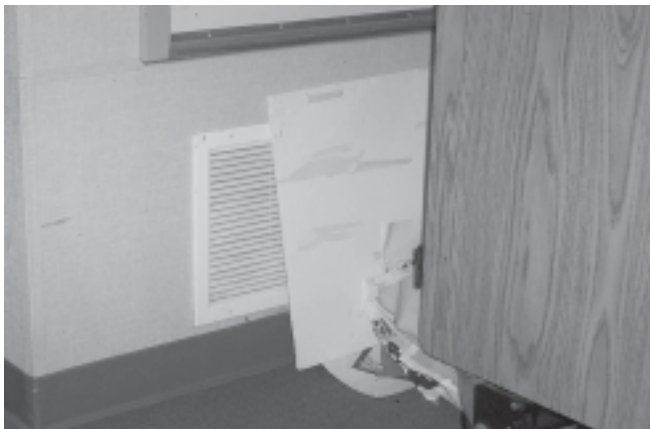
US EPA funded indoor air quality assessments at seven schools in the Ravenswood City School District. Blocked vents were one of several problems detected that can contribute to poor air quality and can worsen asthma.
